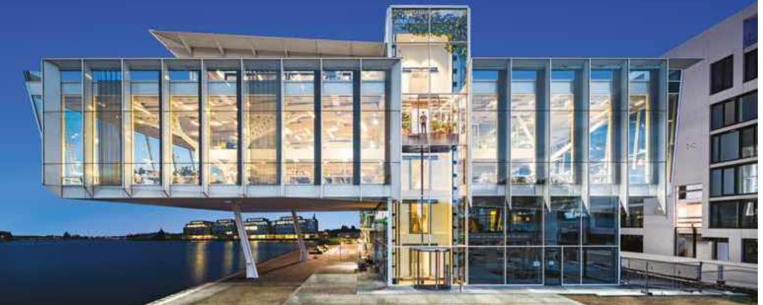
Exterior view of Amvest headquarters. At the heart of the building is the slow elevator that doubles as a movable meeting room. © Studio de Nooyer - V2com
